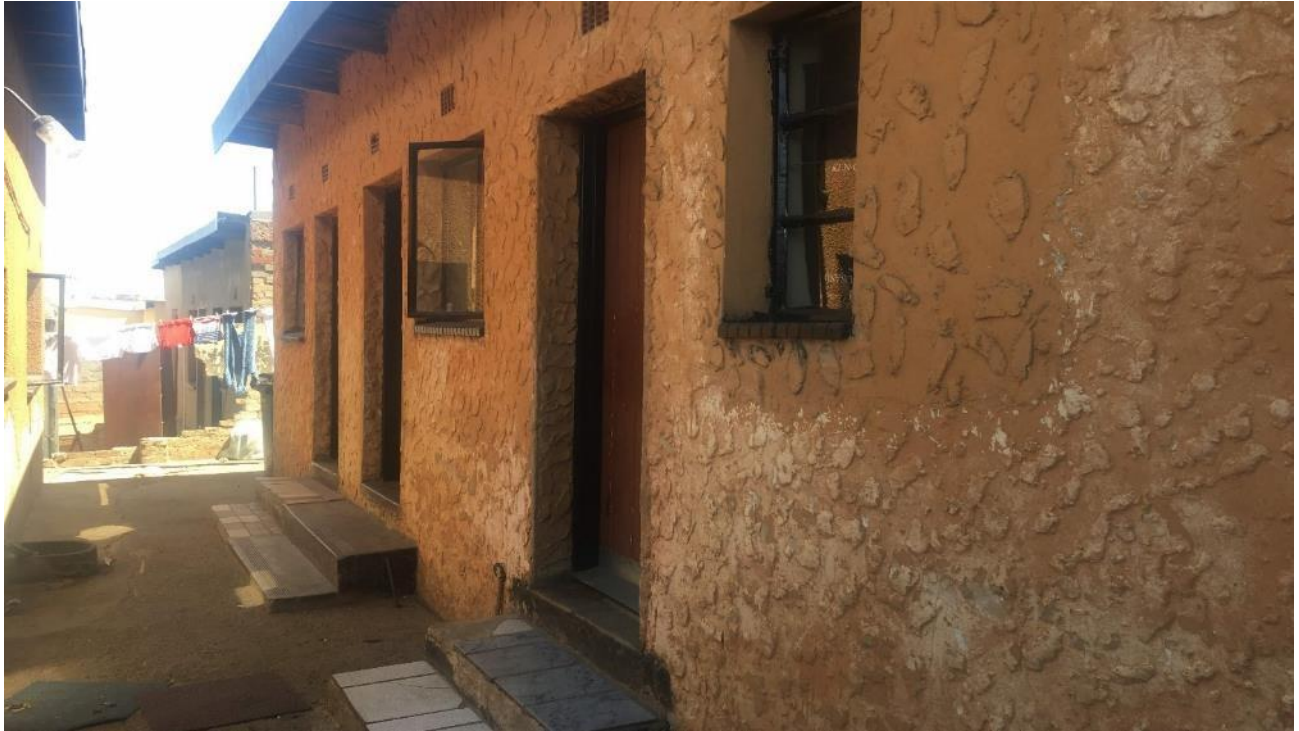
Figure 24: Brick and mortar backyard structures (Photo by Chabalala, 2019)
