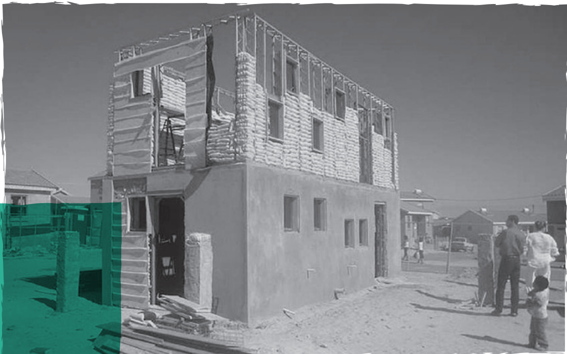
10 x 10 Sandbag housing, Mitchells Plain, Cape Town. Image courtesy of Wieland Gleich – ARCHIGRAPHY.com
