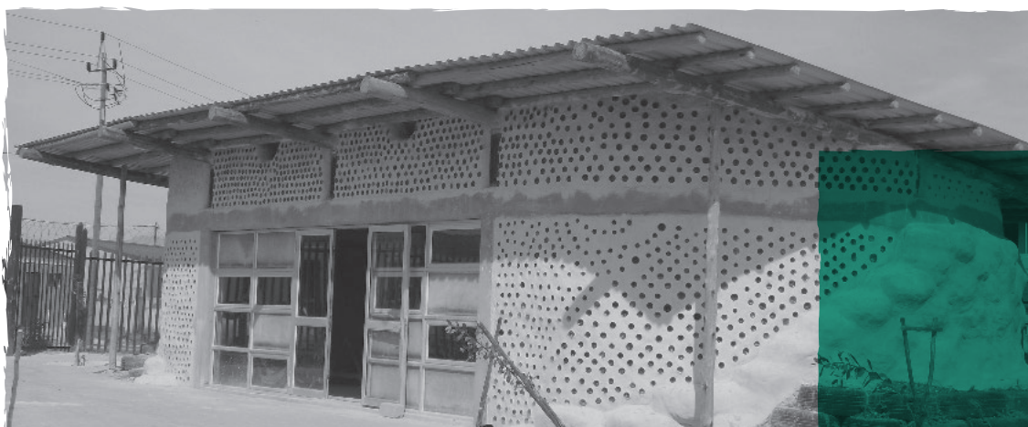
Delft Early Childhood Development Centre. Image courtesy of City of Cape Town, Architectural Unit.
